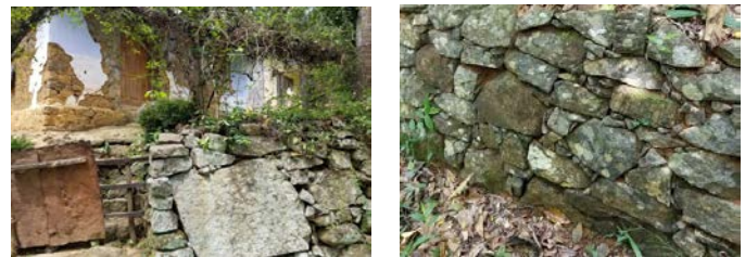
Fig.7. Retaining Walls. Source: Author.
